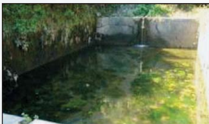
Figure 11: Water tank constructed during the project
